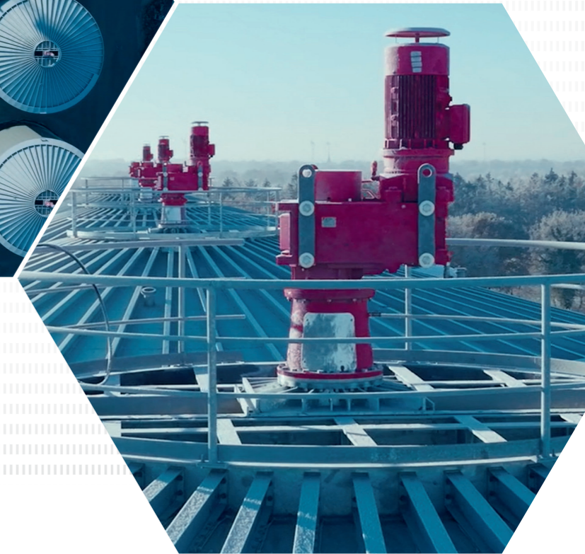
Drives for Europe's largest biogas fermenter In a gigantic biomethane plant in Friesoythe in Lower Saxony, the agitators are operating with robust industrial gear units from NORD's MAXXDRIVE® series.
